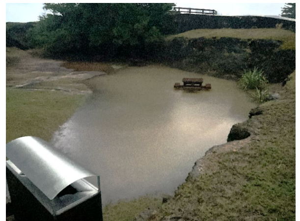
January 2026 flooding at Lime Kiln Picnic Area
