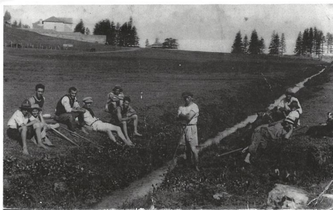
Prior to mechanical clearing of the channels, the channels were manually cleared and significantly narrower. Image to the left shows the channel (and workers) in the lower section of Watermill Valley, with Pier Street bridge visible in the background, far right. (Image undated but possibly Depression-era work? Courtesy Robin Adams)
