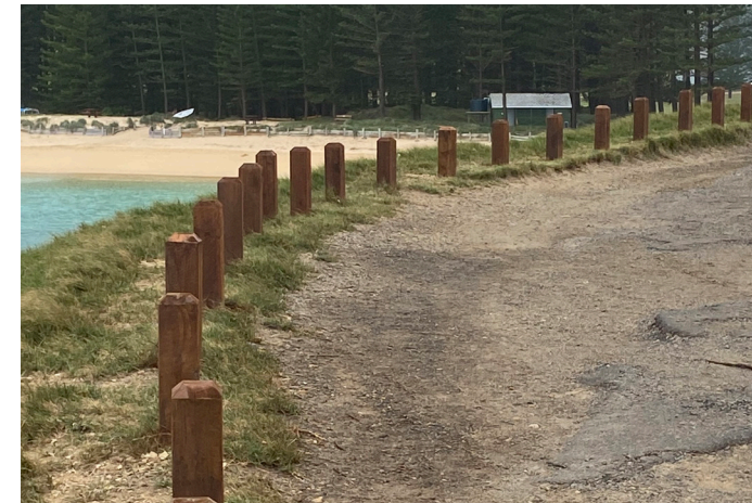
FIGURE 72. EXISTING ROAD NEAR EMILY BAY SHORE
