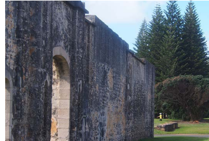
FIGURE 112. PRECINCT WALLS AT THE PRISONER'S COMPOUND
