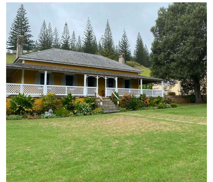
FIGURE 47. NO.10 QUALITY ROW HOUSE AND GARDEN
