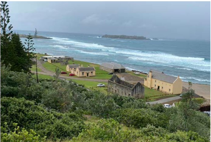
FIGURE 115. VIEW OF KINGSTON PIER FROM FLAGSTAFF HILL
