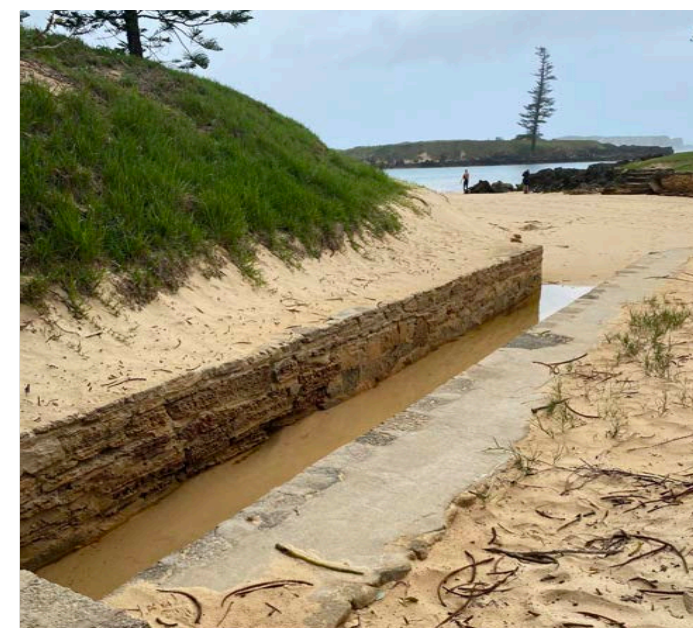
FIGURE 54. DISCHARGE POINT OF WATERMILL CREEK TO EMILY BAY
