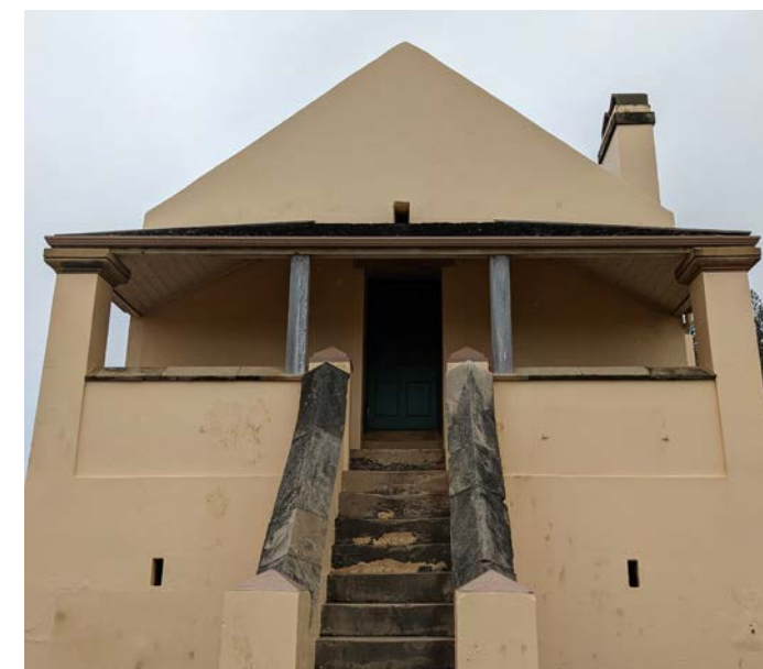
FIGURE 65. PIER STORE EXTERNAL STAIR
