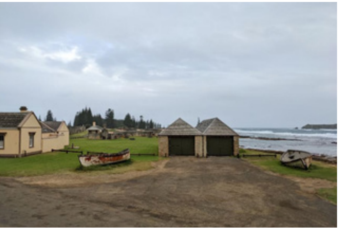
FIGURE 84. BOAT SHED AT KINGSTON PIER
