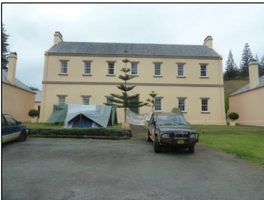
Figure 31: OMB Main Building
