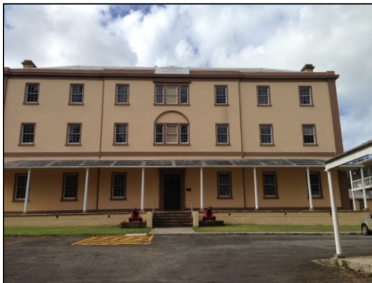
Figure 27: NMB Main Building
