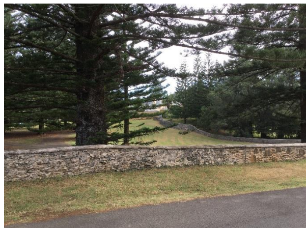
Figure A3.12 View into Government House grounds, showing mature Norfolk Island pine (harming the physical fabric of the stone wall) and smaller self-sown pine (right). (Source: Context + GML 2018)
