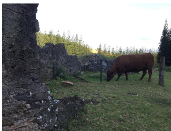
Figure A2.6 Livestock in close proximity to historic fabric (walls and standing structures) presents risks of physical damage to significant fabric. (Source: GML + Context 2018)
