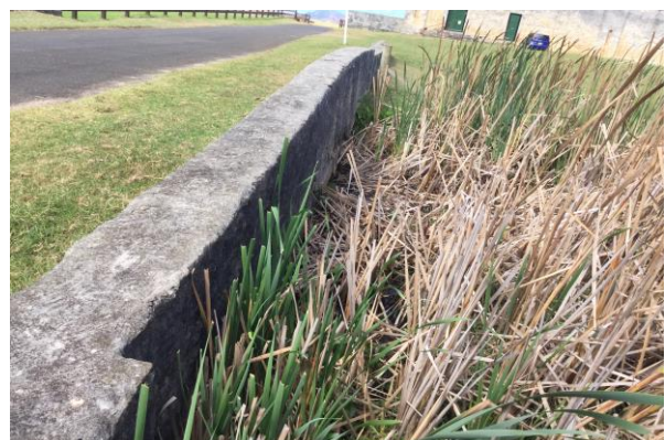
Figure A4.4 Reeds damming and slowing water flow, contributing to saturation of soil on Kingston Common (Bounty Street Bridge shown). (Source: Context + GML 2018)
