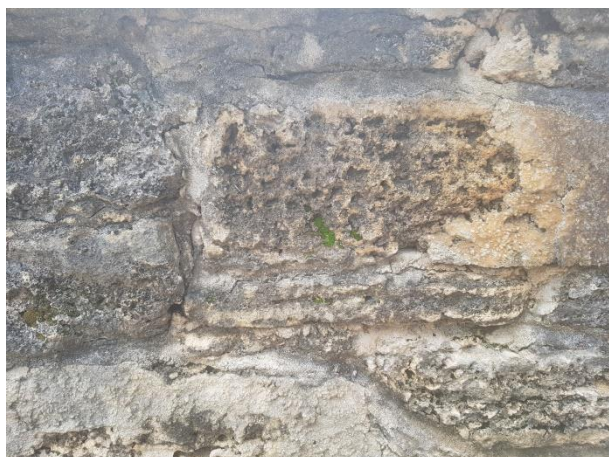
Figure 65 View of calcarenite showing its porous properties
