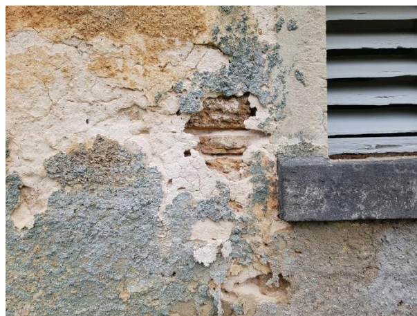
Figure 66 View of calcarenite showing inappropriate surface render
