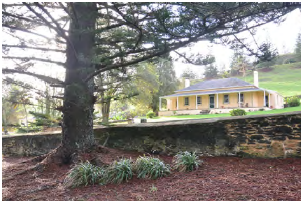
Photograph 14 (above). Garden wall damage along Quality Row caused by roots of neighbouring pines.
