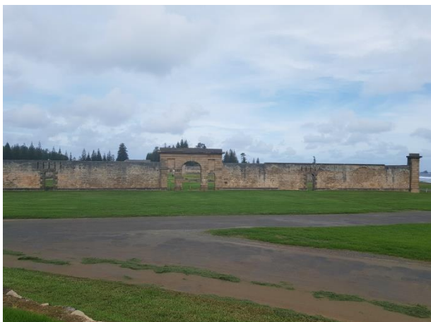
Figure 33 View of New Gaol showing perimeter wall
