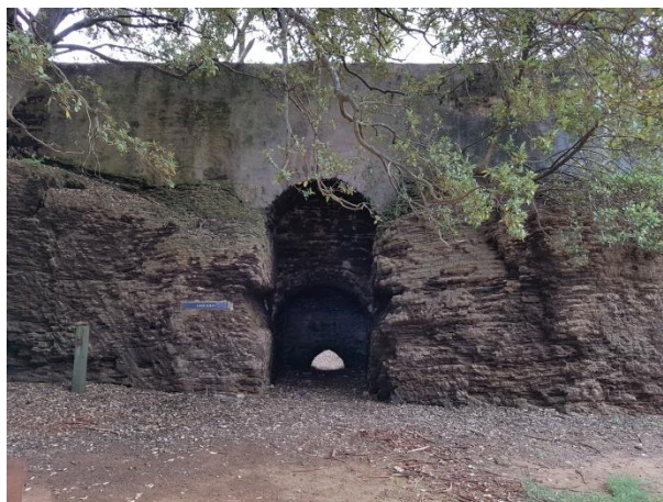
Figure 50 View of Lime Kiln
