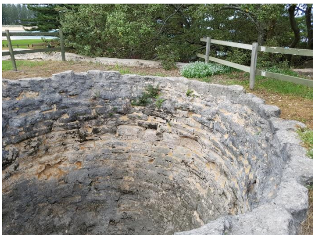
Figure 51 View of Lime Kiln and grotto like remains
