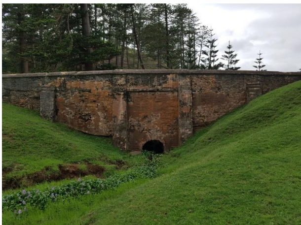
Figure 61 View of Bloody Bridge looking west showing drainage to Cemetery Bay
