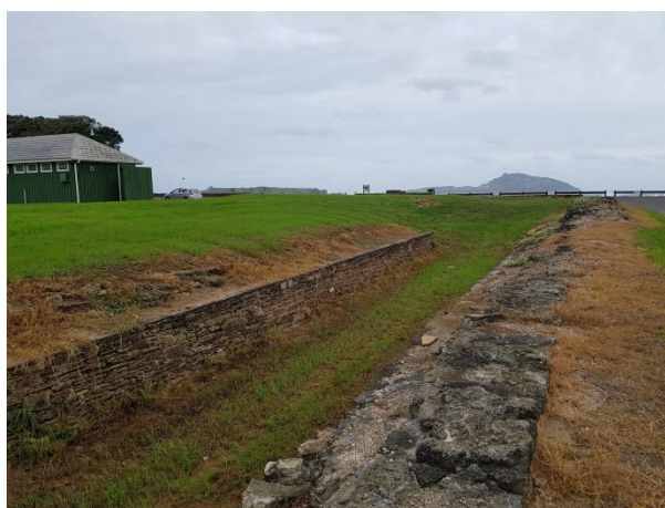
Figure 36 View of Changing shed showing ruins along Bounty Street
