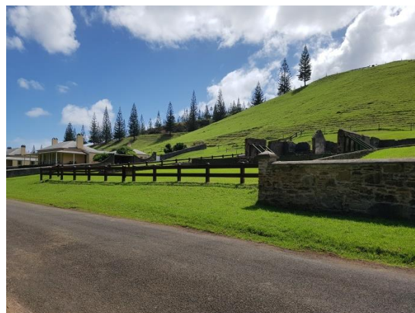
Figure 23 View of Quality Row showing building ruins and steep cleared hills as a backdrop
