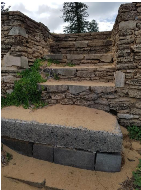
Figure 45 Detail view of stone sea wall at Slaughter Bay
