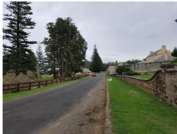
Figure 21 View of Quality Row looking west showing stone fencing, kerbed and free draining road, grassed footpaths
