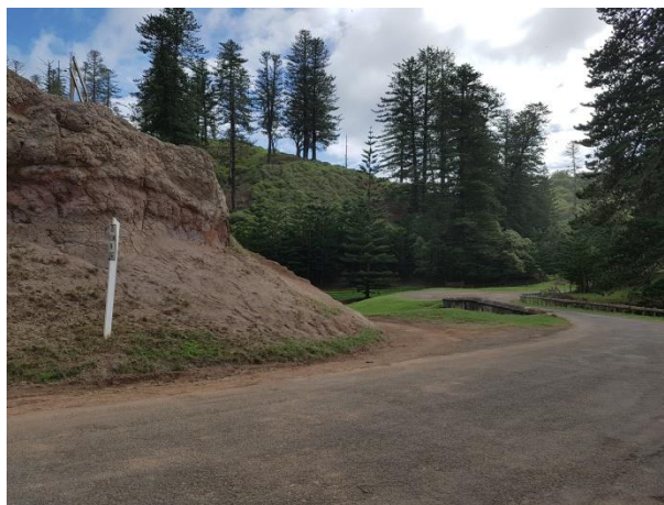
Figure 64 View of Bloody Bridge looking north showing area steep slopes
