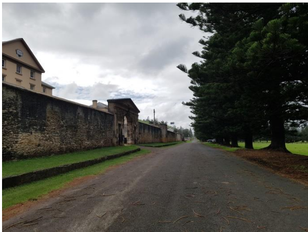
Figure 20 View of Quality Row looking east showing Commissariat Store, perimeter walls and formal plantings of Norfolk Island Pines
