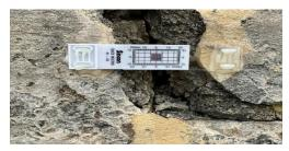
Tell-tale slides (pictured) have been installed on several heritage buildings to monitor cracks in the stone work. This is a part of regular cyclical maintenance and helps in identifying changes in the condition of buildings.
