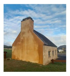
We're also testing a lime mix designed for harsh marine environments to cope with the wall's exposed position. To further protect the base of the wall, we've added a hand-cut stone V-drain from local calcarenite and set with lime mortar, this will help redirect surface water.
