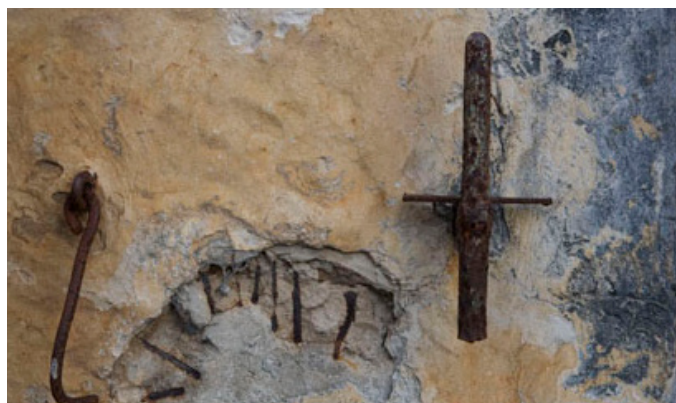
Typical corrosion presentation of embedded metals.
