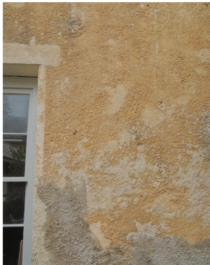
A range of treatments at No. 10 Quality Row, note the whitewashed boarder to the lintel and window reveal.
