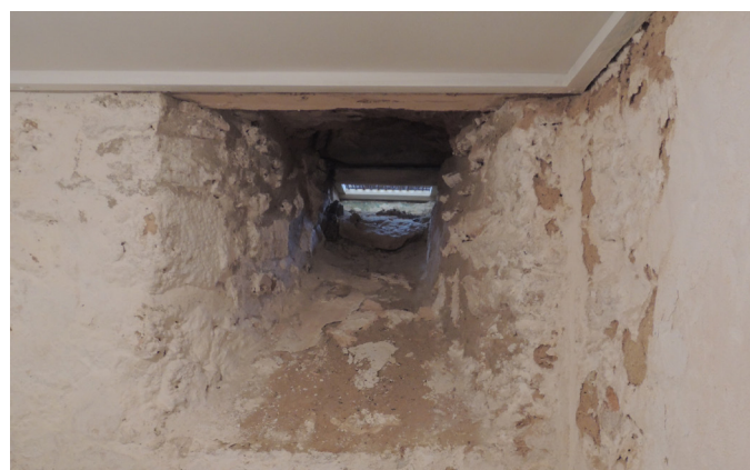
Limewash applications to the Government House Cellar are performing well by comparison.
