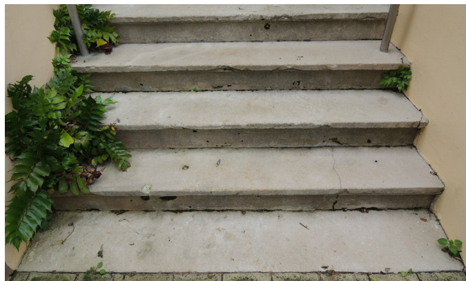
Stones to Government House demonstrate signs of bleaching and discolouration from cleaning.
