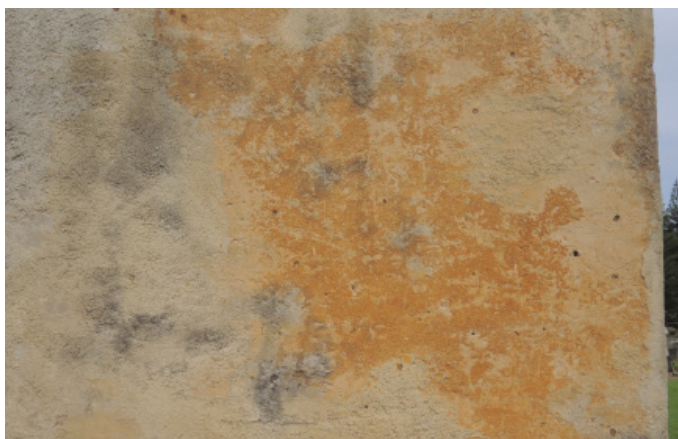
Extant renders and harling to the outbuildings of No. 10 Quality Row. Source: Purcell.
