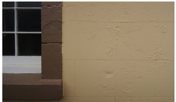
The Settlement Guardhouse exterior with significant bubbling and failure of acrylic paint coatings.
