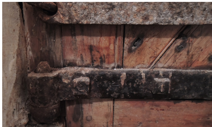
Deterioration of Cellar door hardware due to corrosion, presenting risk to adjacent fabric.
