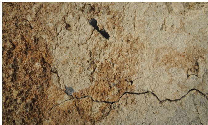
Evidence of original renders and harling at No. 10 Quality Row.
