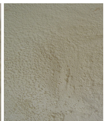
Paint failure within the Prisoner Barracks Museum trapped salt crystallisation.
