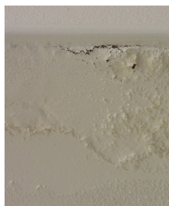
Paint failure to the Royal Engineers is expressed both internally and externally.
