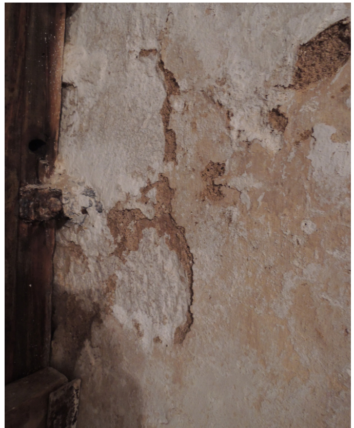
The Government House cellar, with limewashed walls shows limited evidence of salt attack adjacent areas of water ingress. Note the different failure mechanism to that of acrylic paint.
