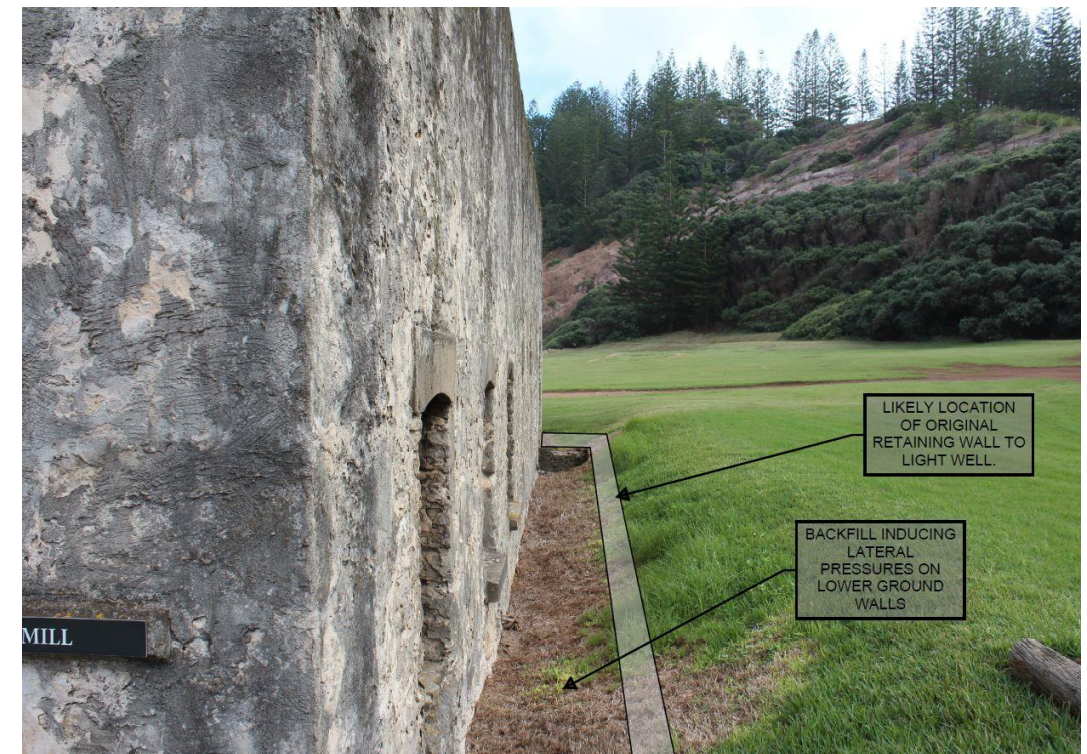
Backfill in light well and location of potential parking.
