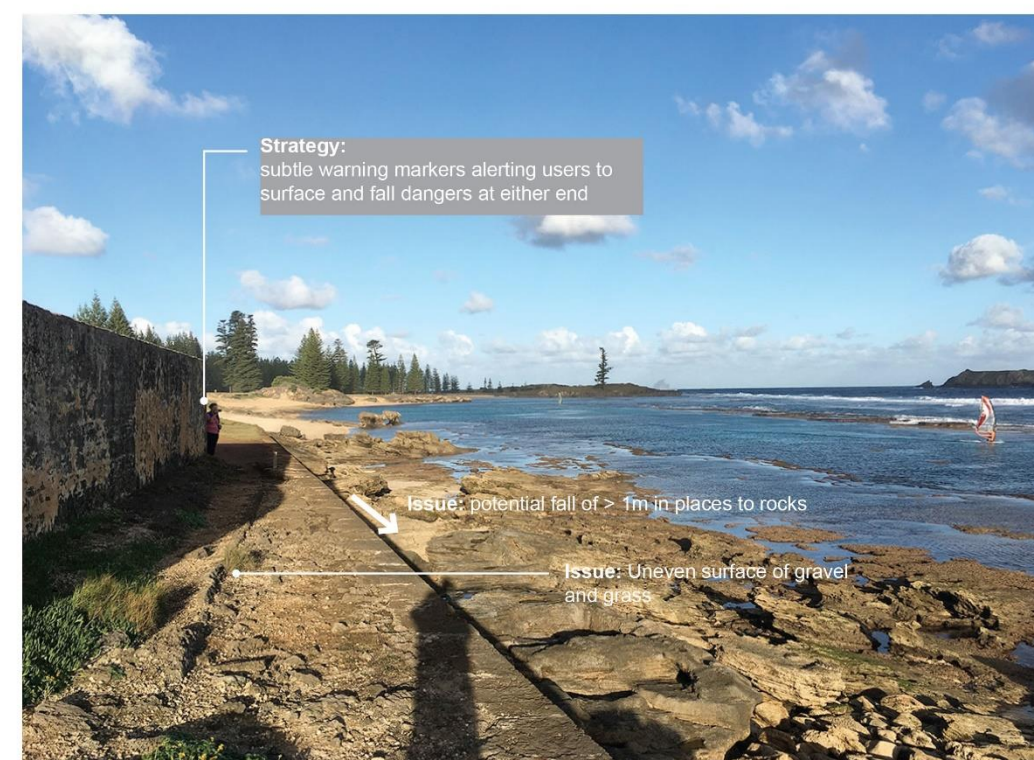
Example of drop off from walking route / accessible areas foreshore near Kingston Pier
