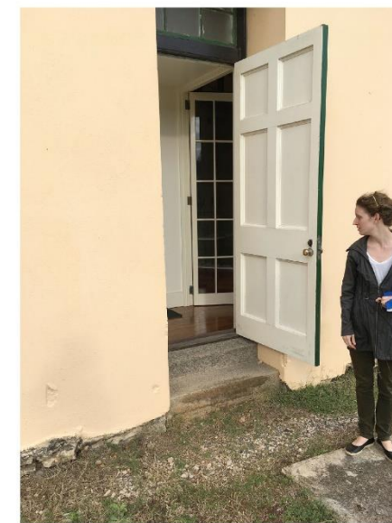
Side entry used for temporary "pop up" disabled / wheelchair access to Sirius Museum
