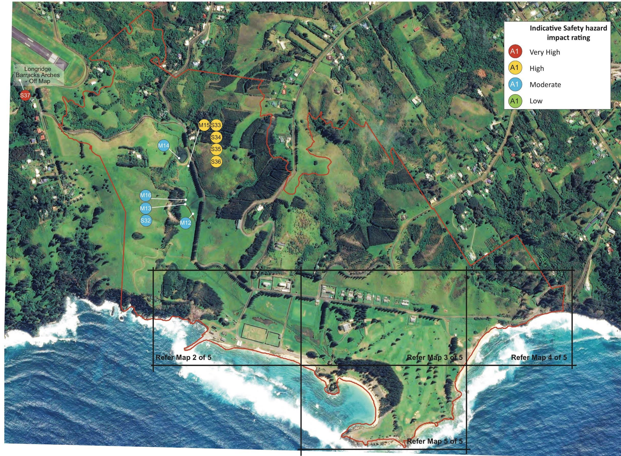
KAVHA Safety Hazard Scoping Study 2018
