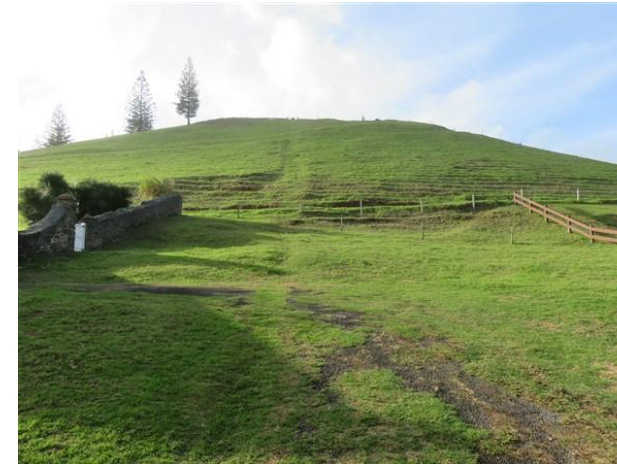
Hill behind Nos 4 and 5 Quality Row showing landslip in the area between the houses.
