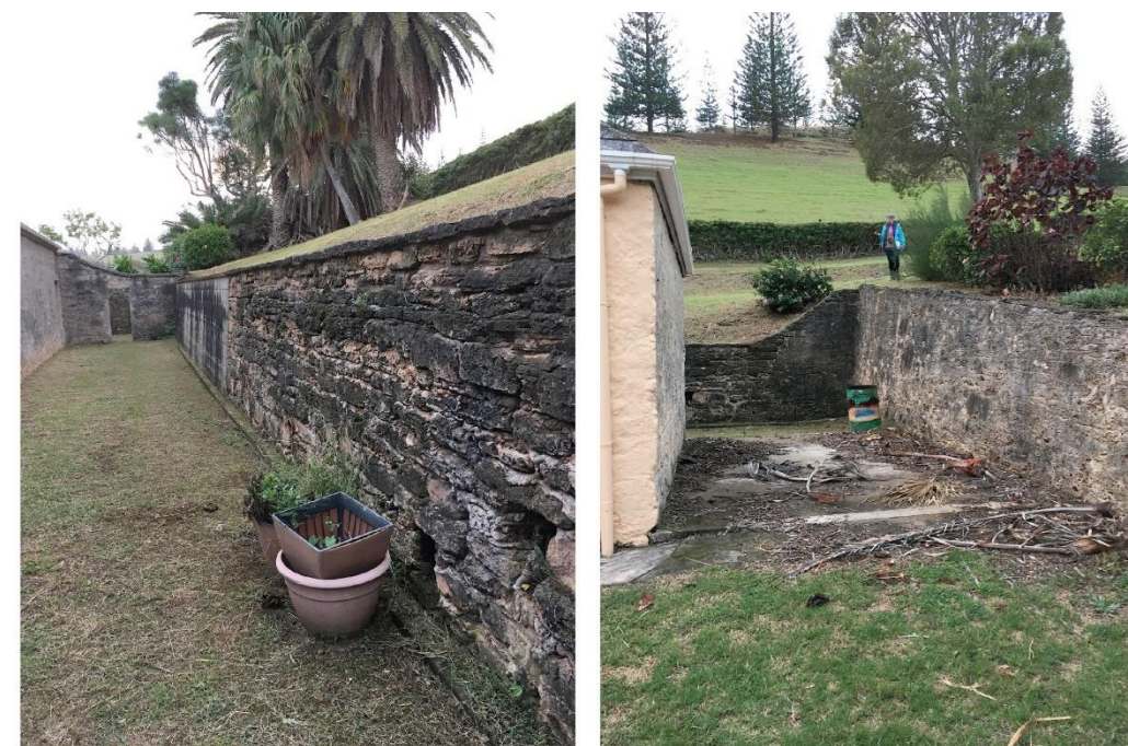
Typical rear wall at No 9 Quality Row
