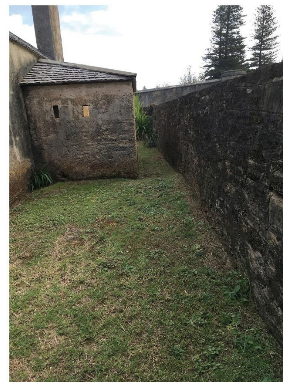
Typical rear wall at No 7 Quality Row
