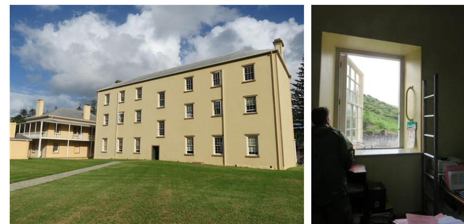
Pull out ladders are fixed to the rear wall of the Old Military Barracks to provide an alternate fire escape. Access to the ladders is through the windows.
