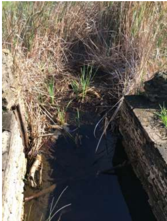
Figure 53 Channel exit blocked by weeds
