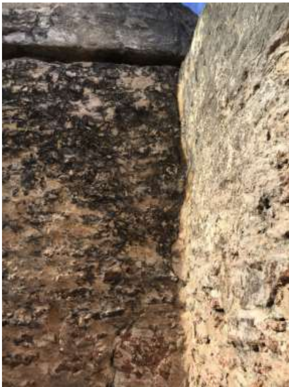
Figure 6 Crack in the gable interior face top
