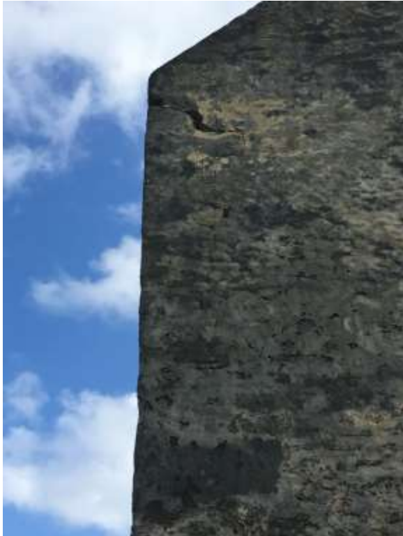
Figure 8 Crack in the gable exterior face
