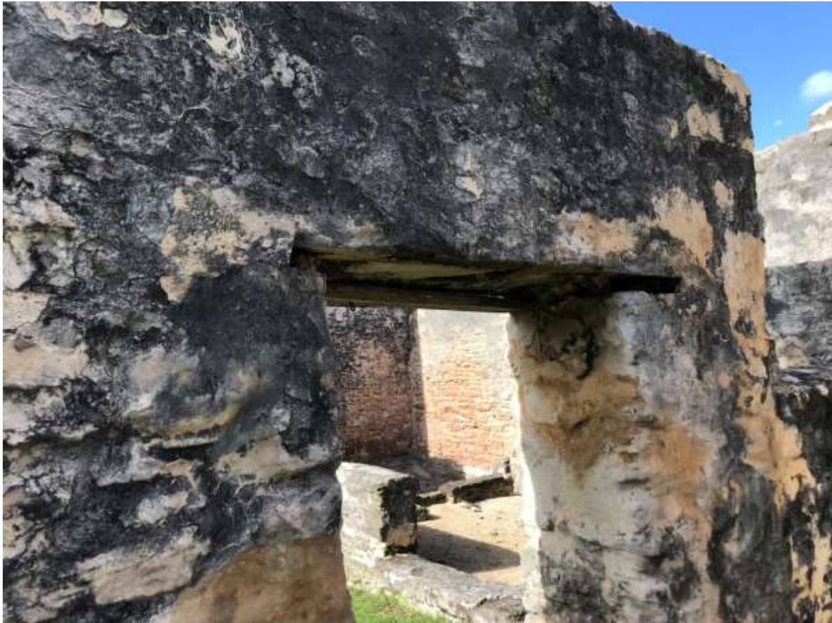
Figure 17 Missing lintel on southern face of doorframe
