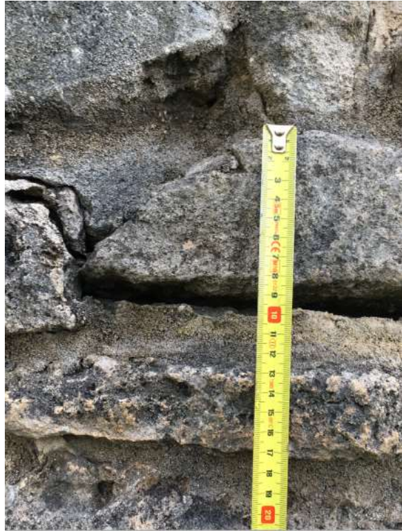
Figure 40 Cracking in the retaining wall
