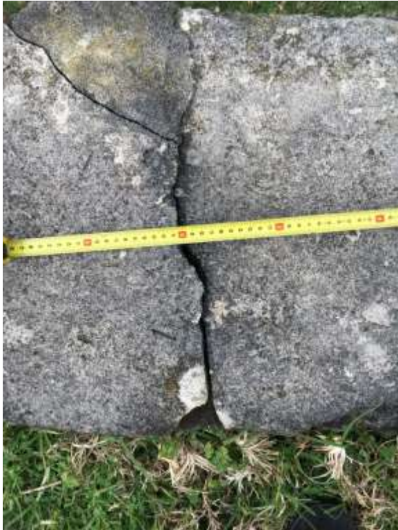
Figure 39 Cracking in top of retaining wall
