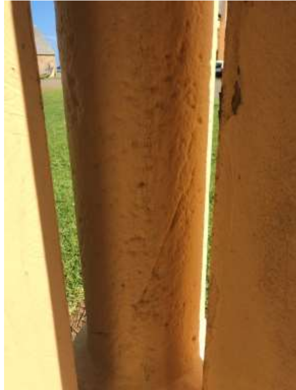
Figure 77 Possible cracking in bottom of southern column
