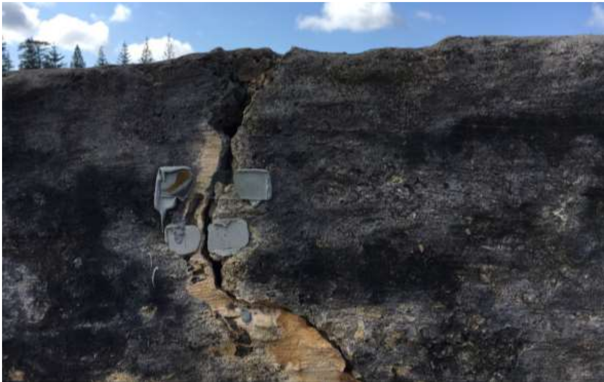
Figure 58 Glass tell-tale on side of crack in the western portal
