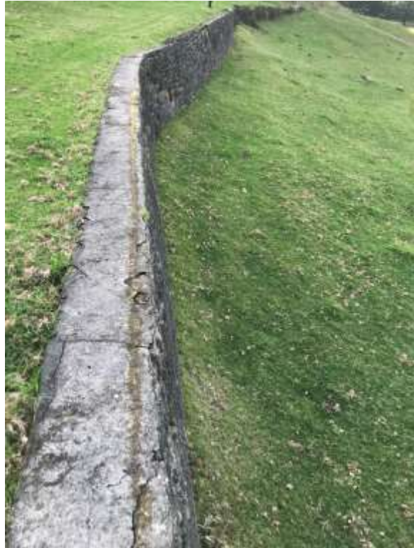
Figure 29 Bulging of retaining wall
