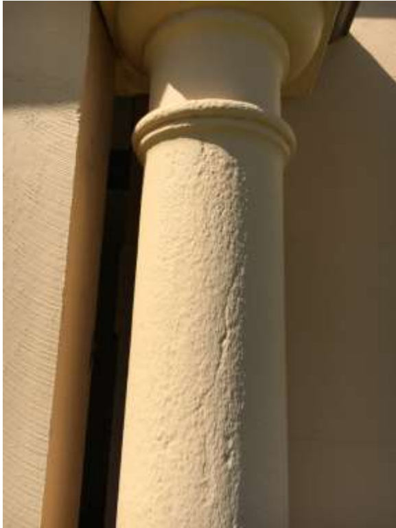
Figure 76 Possible cracking in top of southern column
