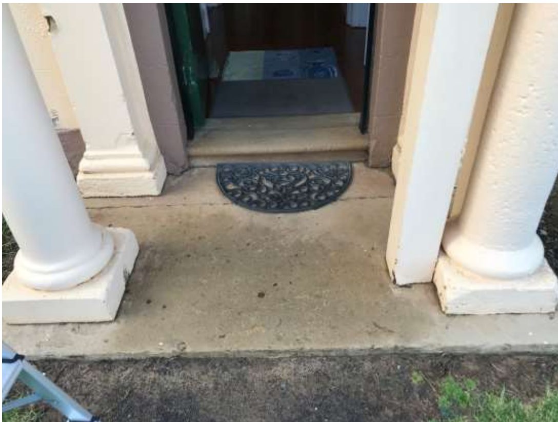
Figure 81 Base Slab of the Portico
