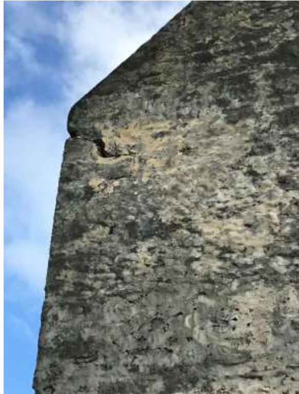
Figure 9 Crack in the gable exterior face
