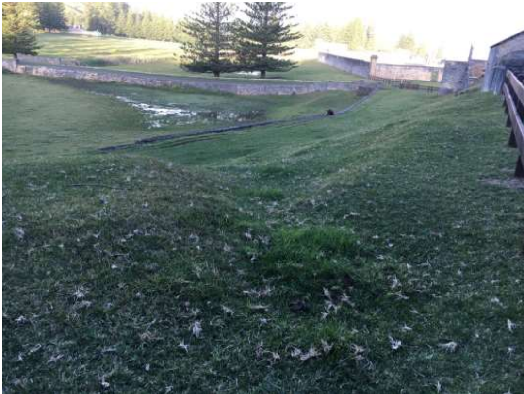
Figure 44 Slope of land funnelling water down into retaining wall from hill behind
