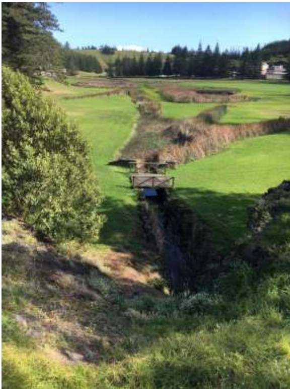
Figure 52 Drain channel overrun by weeds
