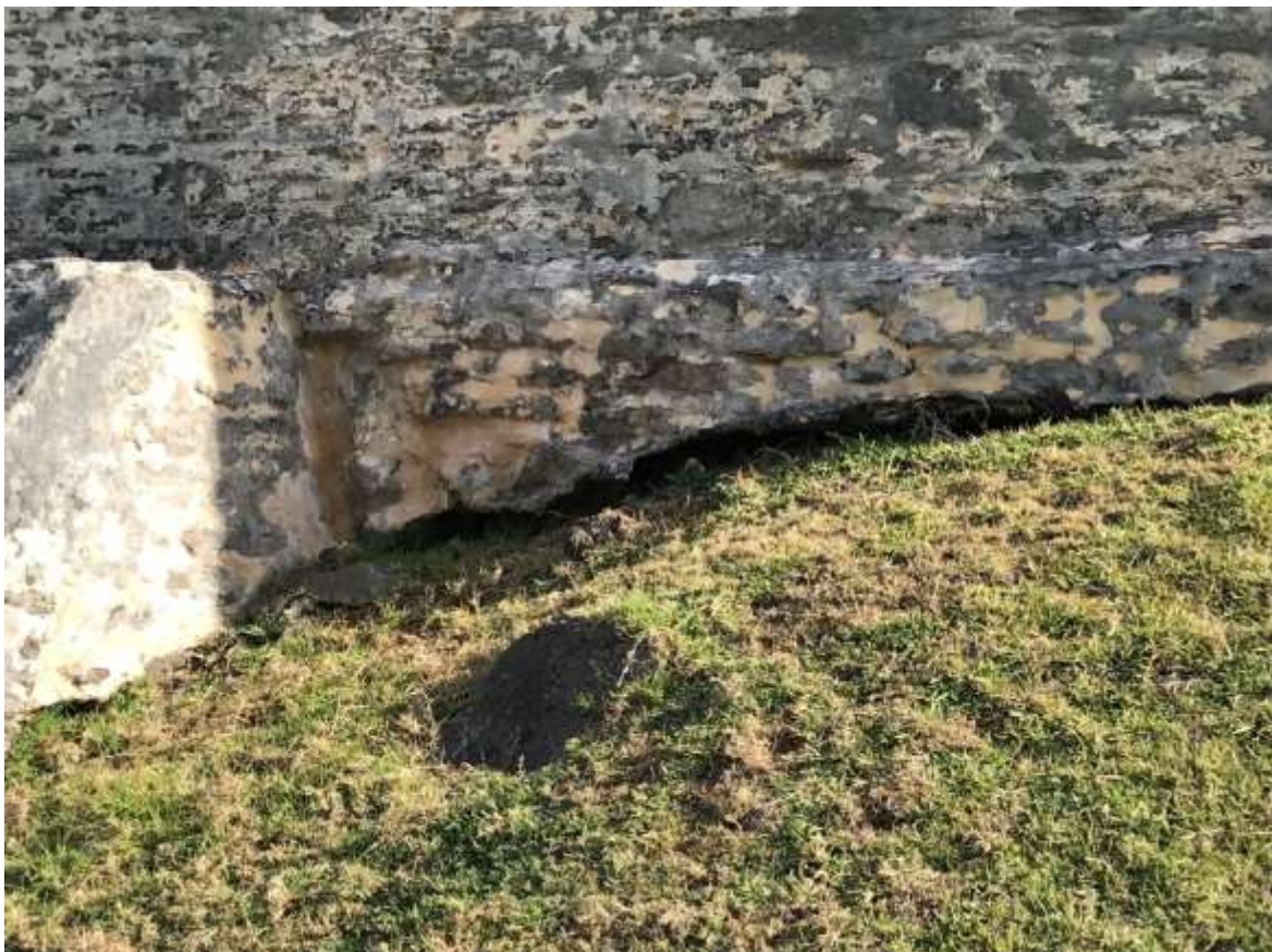
Figure 10 Lowered ground line to the northern exterior of gable
