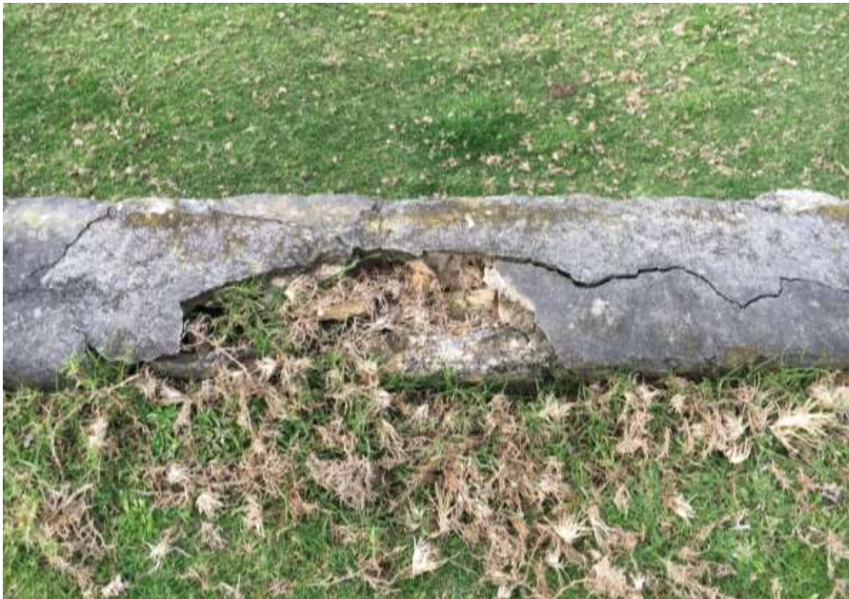
Figure 41 Damage to top of retaining wall
