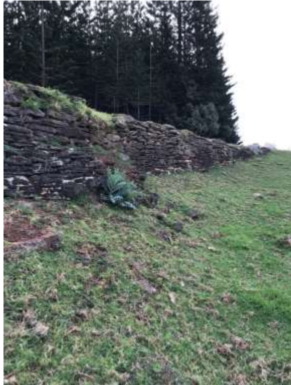
Figure 43 Portion of retaining wall without mortar
