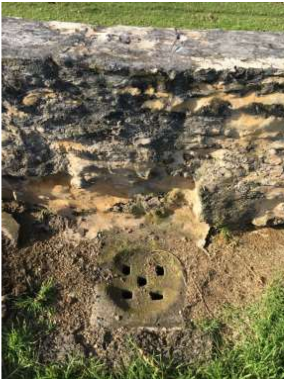
Figure 15 Drain below the retaining wall
