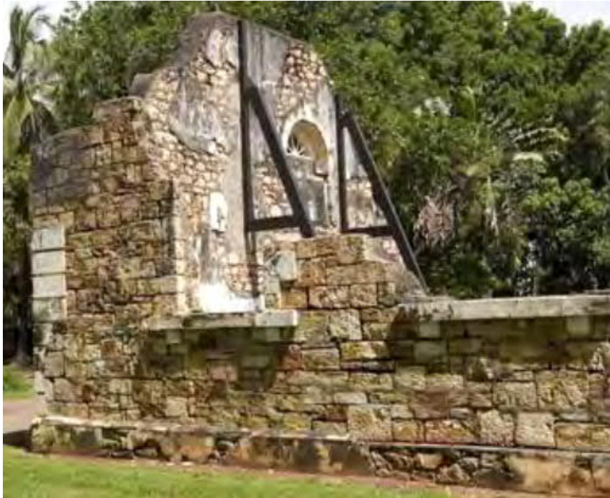
PHOTO OF PROPOSED GABLE BRACING
