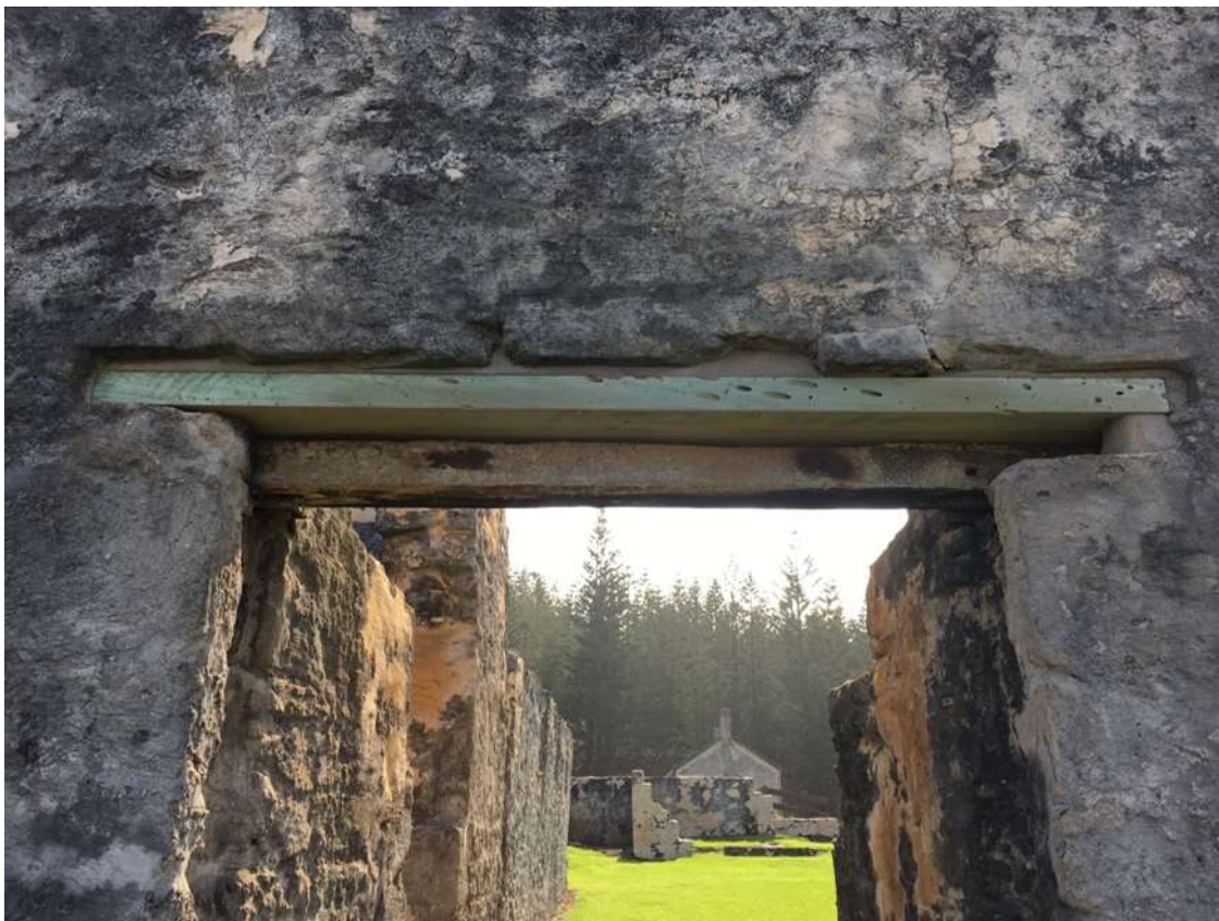
Figure 25 Replaced timber lintel on eastern entrance into the Civil Hospital
