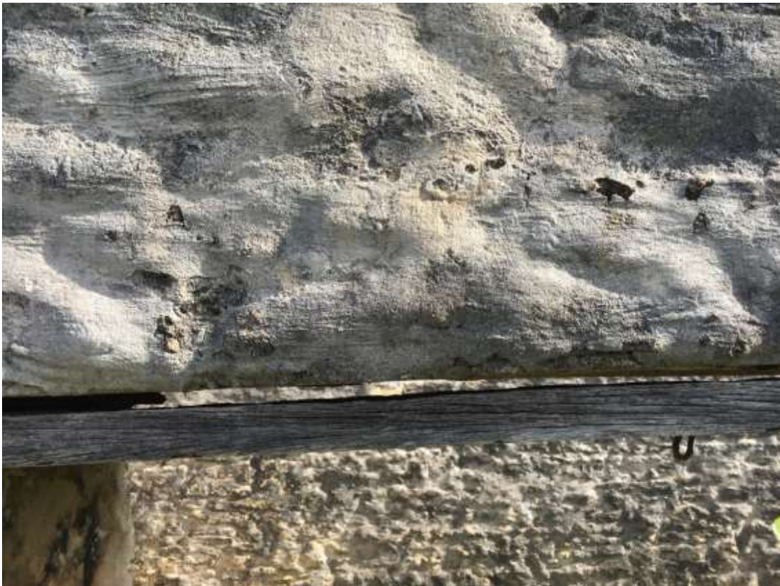
Figure 20 Space between stone doorframe and existing timber lintel on northern face
