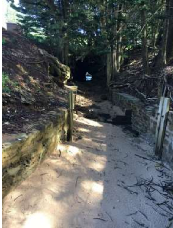
Figure 55 Drain tunnel filled with sand and debris
