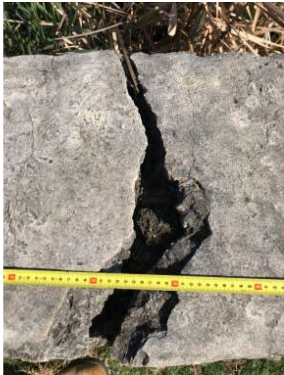
Figure 57 Crack in the western portal
