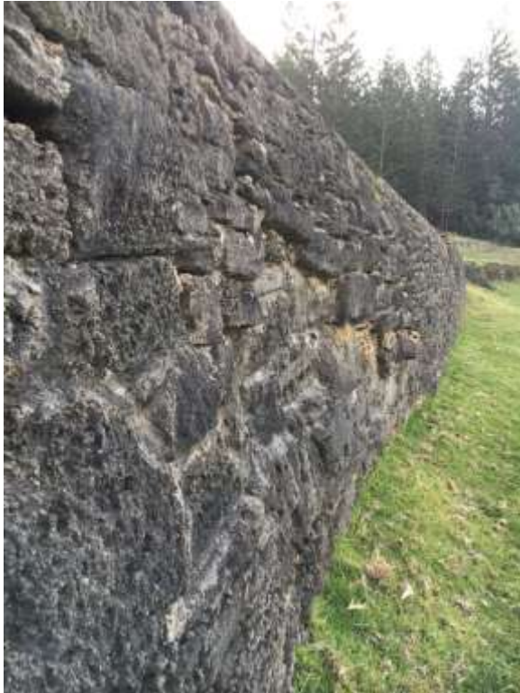
Figure 28 Bulging of retaining wall
