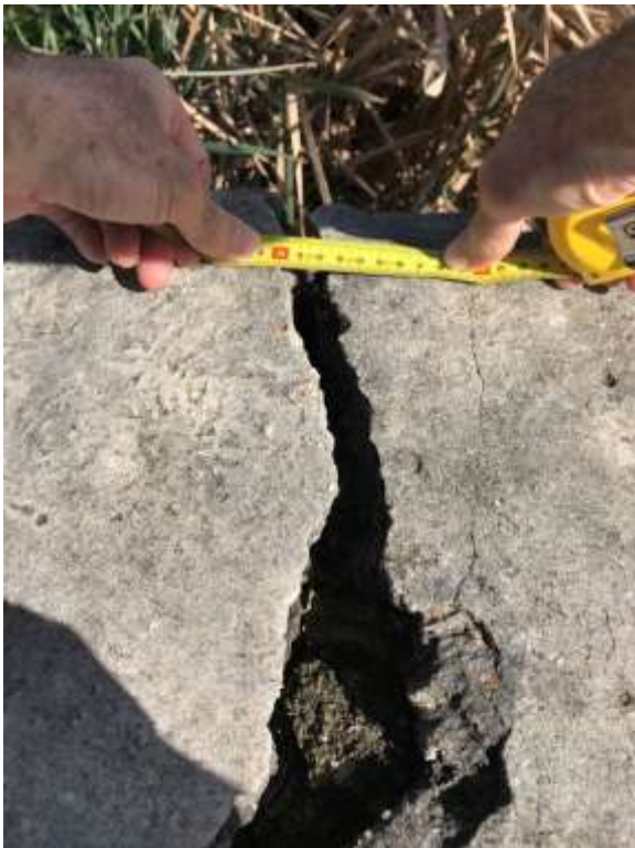
Figure 56 Crack in the western portal
