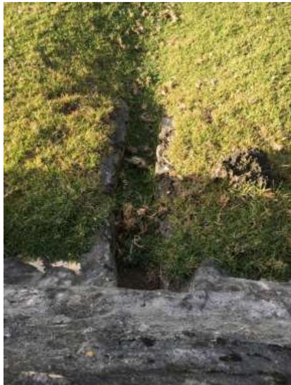
Figure 16 Drain run out below the retaining wall
