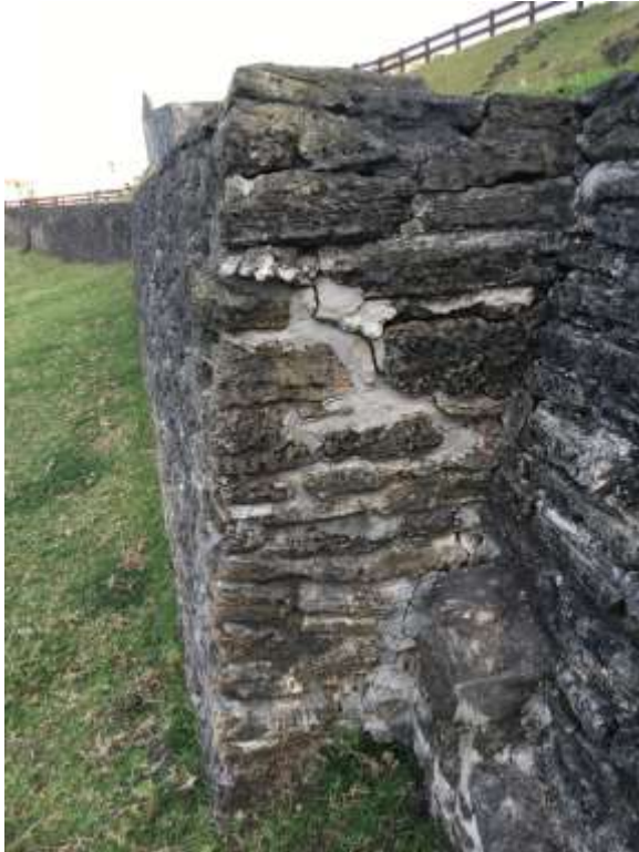
Figure 42 Cracking and gaps in the mortar
