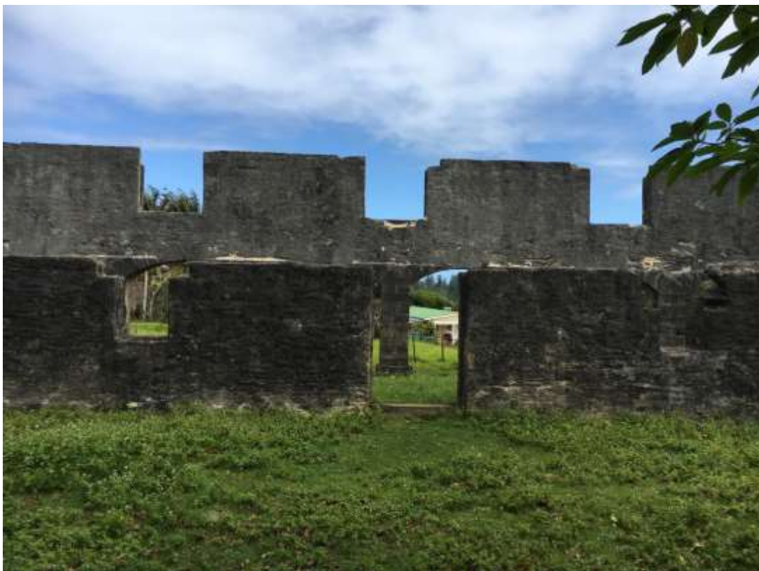
Figure 69 Longridge Barracks lack of structure behind wall from rear of wall
