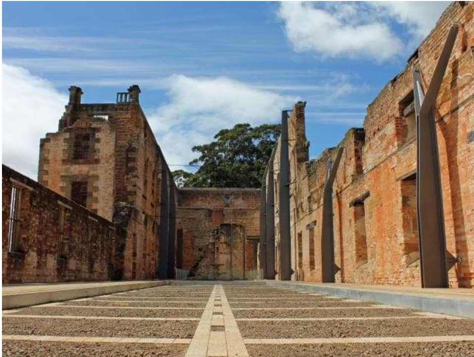
Figure 70 Bracing for walls at Port Arthur Penitentiary (Mercury, 2014)
