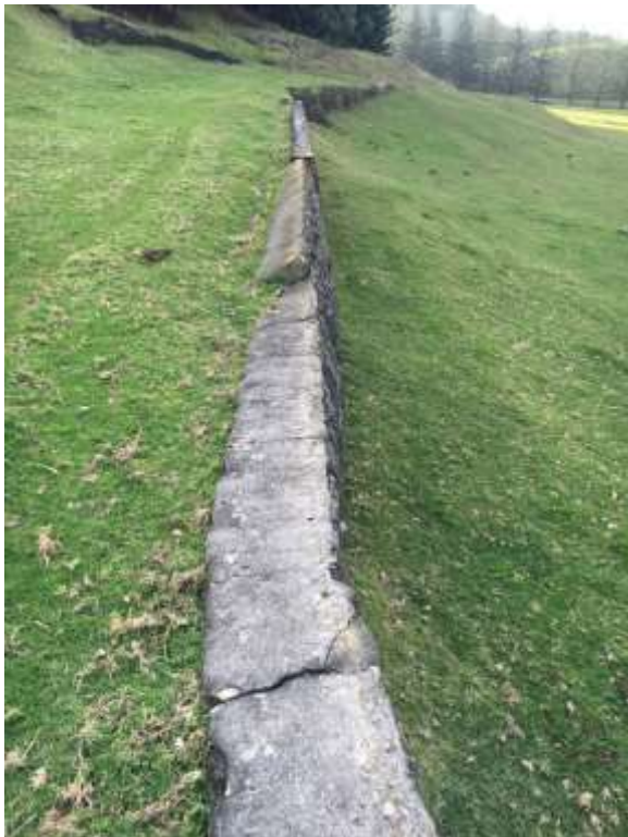
Figure 30 Rotation of the top of the wall
