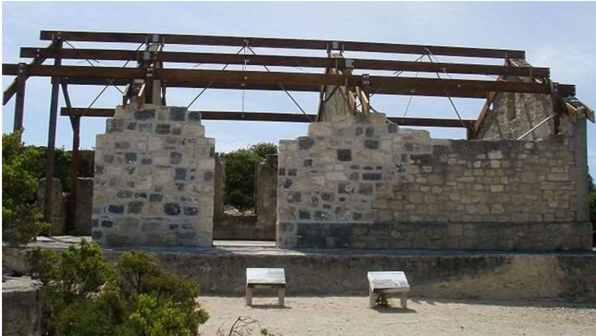
Figure 23 Weir Cove storeroom after restoration and reconstruction (Department of Environment, Water and Natural Resources)
