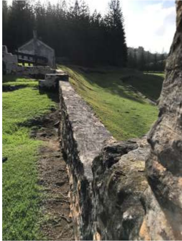
Figure 14 Interior of the top of the retaining wall
