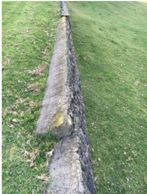
Figure 31 Collapse of top of wall back on itself
