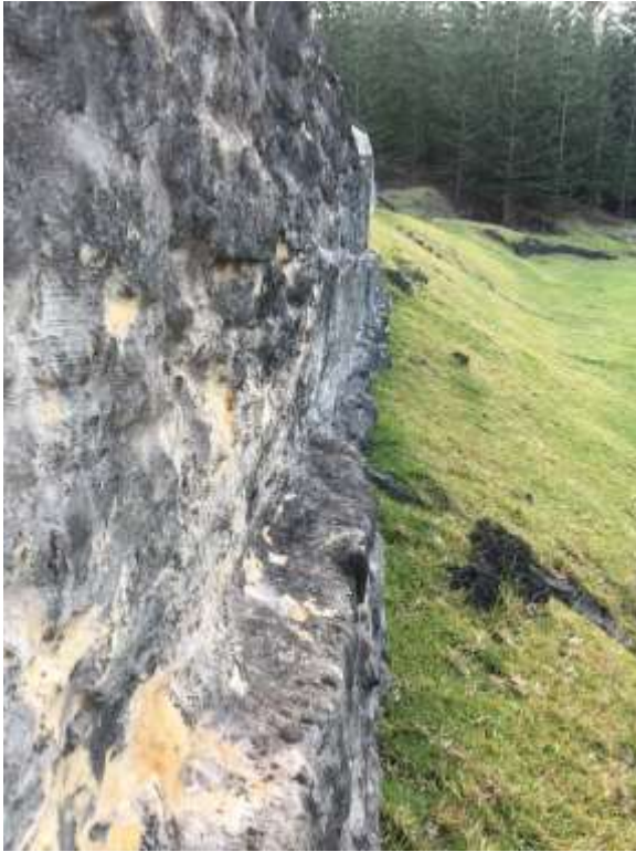
Figure 13 Exterior step out of retaining wall base
