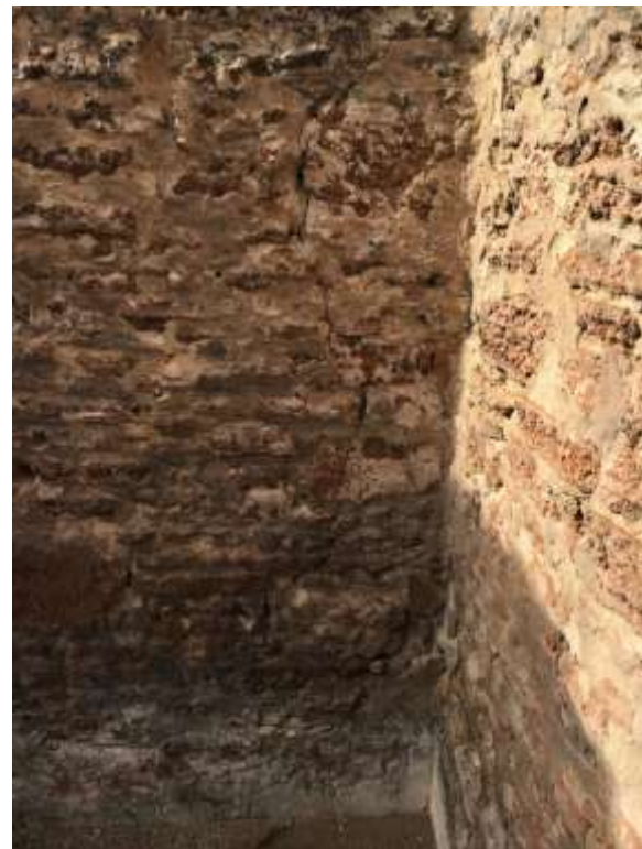
Figure 7 Crack in the gable interior face bottom
