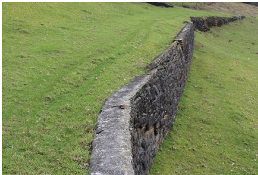
Figure 3 (left) – Bulging retaining wall below Civil Hospital [Source: GML] and Figure 4 (right) – Drain locations in the retaining wall [Source: AECOM]
