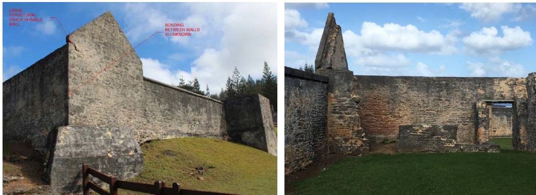
Figure 1 (left) – Northern gable of the Civil Hospital showing structural crack [Source: GML] and Figure 2 (right) – Civil Hospital ruins [Source: AECOM]
