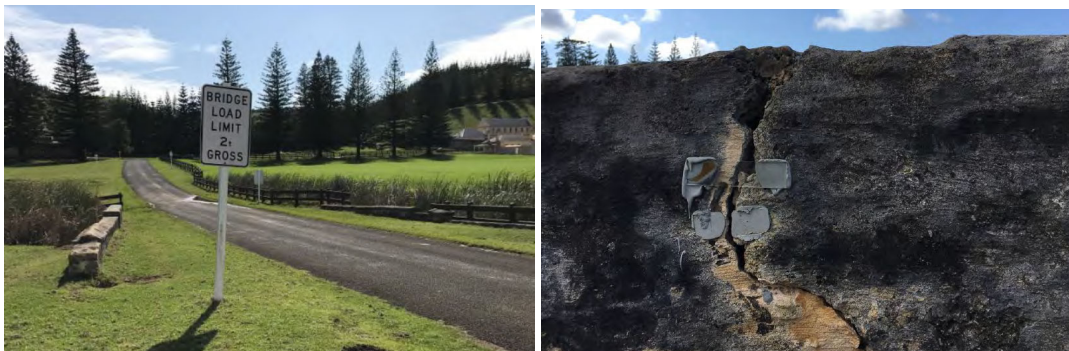
Figure 5 (left) – Bounty Street Bridge and Figure 6 (right) – crack in the western portal [Source: AECOM]
