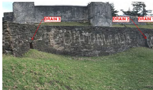
Figure 3 (left) – Bulging retaining wall below Civil Hospital [Source: GML] and Figure 4 (right) – Drain locations in the retaining wall [Source: AECOM]
